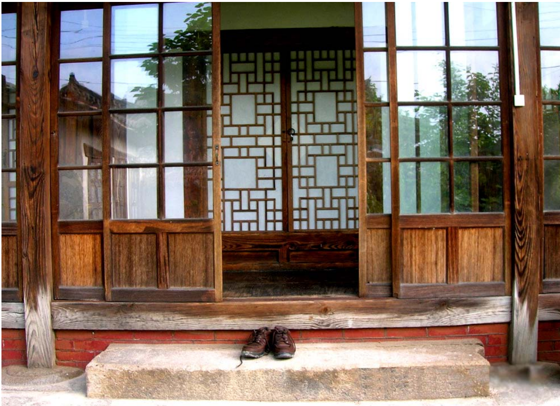
On-Dol Heating System photo by Joseph Rome
