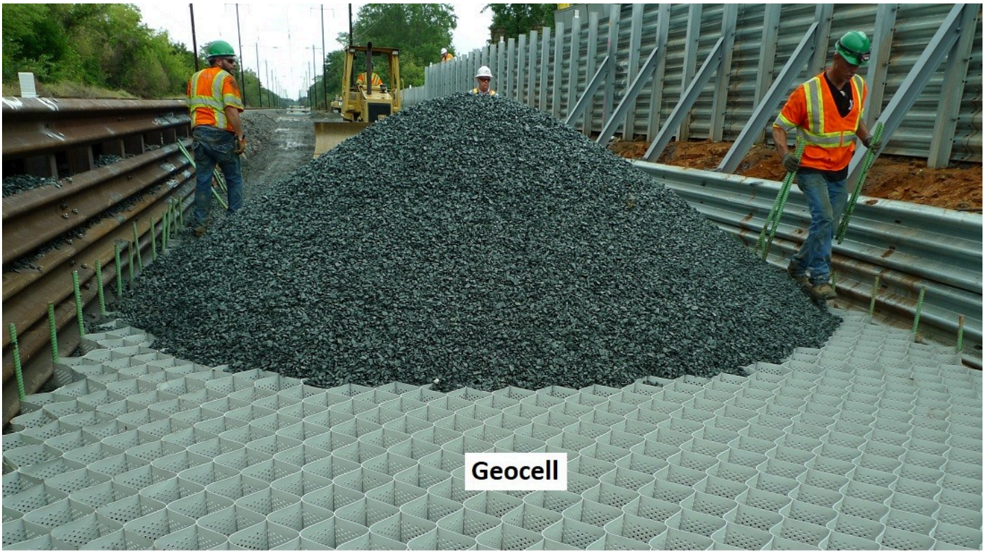
Amtrak's track construction using ballasts and geocells
