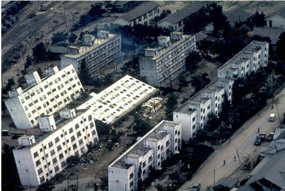
Fig. 3. Overturned buildings due to liquefaction, Niigata, 1964
