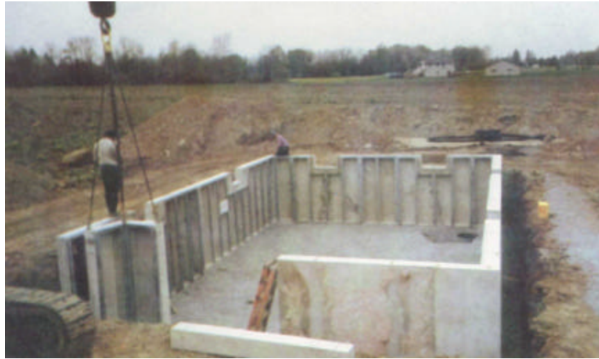
Precast basement panels, in field assembly
