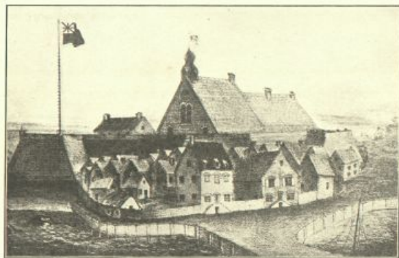
FORT AMSTERDAM AND THE FIRST BRICK DWELLINGS ERECTED IN THE CITY
