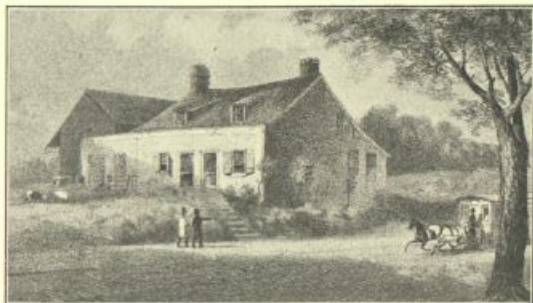
OLD HOPPER HOUSE, 2D AVENUE AND 83D STREET
