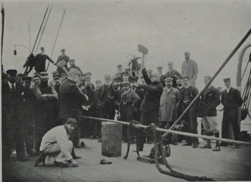
"THE FINAL SPLICE."
