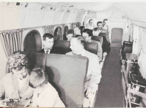
Vertol Cabin Interior
