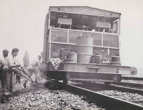
Maintenance of way operations are streamlined by utilization of 27 power-ballasting machines like the one shown above. Also important
