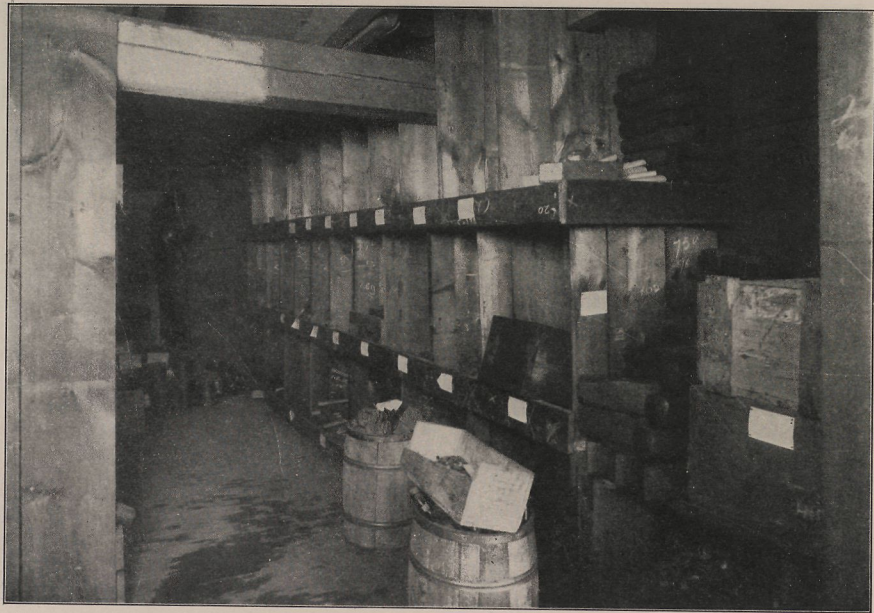
PHOTO. 7.—INTERIOR VIEW—OLD STOREHOUSE—24TH STREET YARD.
