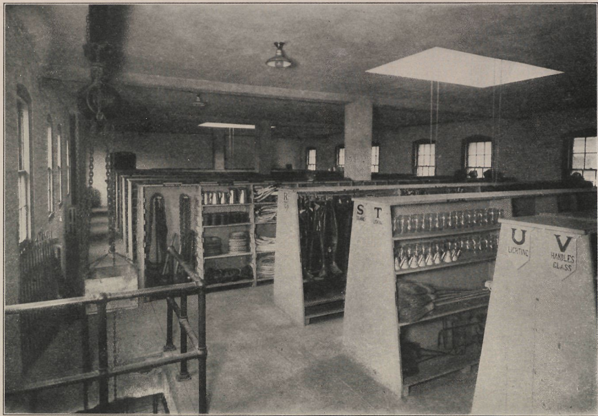
PHOTO. 8.—INTERIOR VIEW—NEW STOREHOUSE—24TH STREET YARD.
