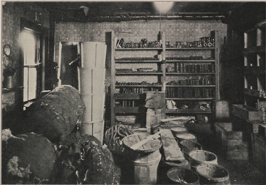
PHOTO. 13.—INTERIOR VIEW OF A LOCAL STOREROOM AT A PUMPING STATION AS IT WAS FOUND BY THE BUREAU OF SUPPLIES WHEN THEY ASSUMED CONTROL.
