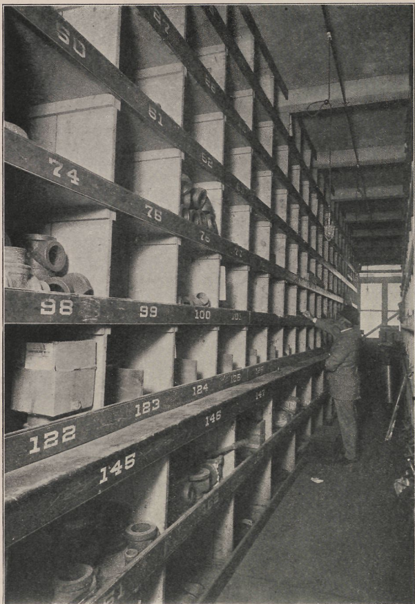
PHOTO. 11.—OLD STORAGE BINS AT RIDGEWOOD.
