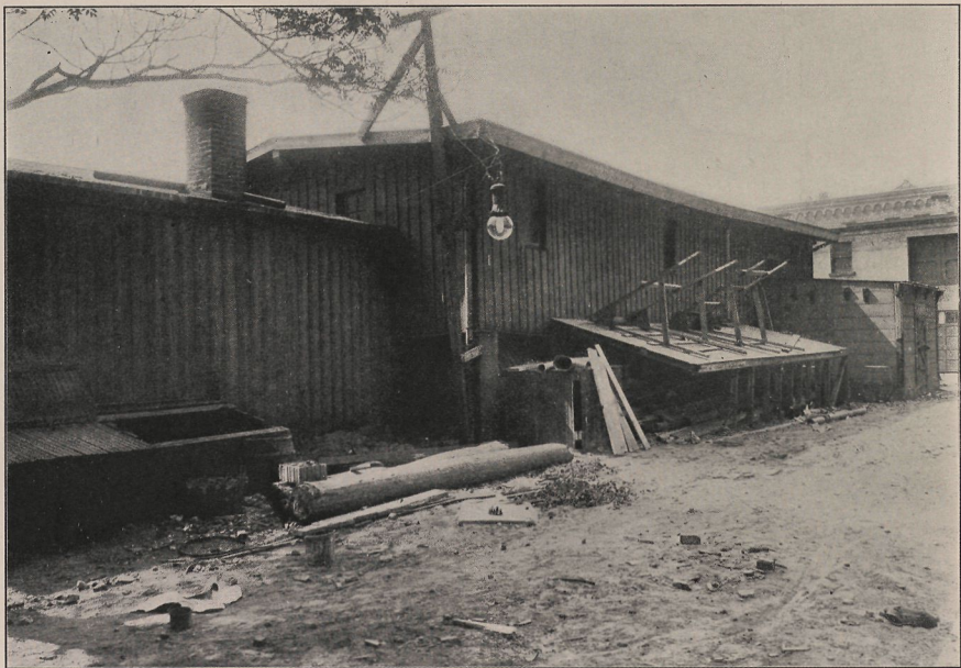
PHOTO. 5.—OLD STOREHOUSE—24TH STREET YARD.
