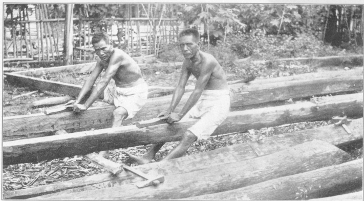
NATIVE CARPENTERS AT WORK.
