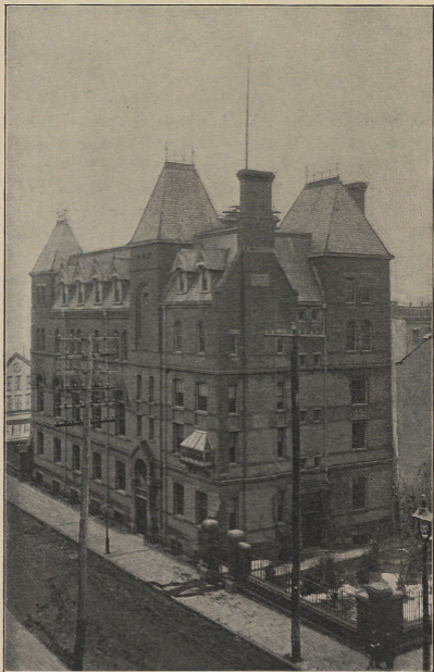
THE EAST SIDE BOYS' LODGING HOUSE AND INDUSTRIAL SCHOOL; ALSO OFFICE OF THE SICK CHILDREN'S MISSION AND FLOWER MISSION.
