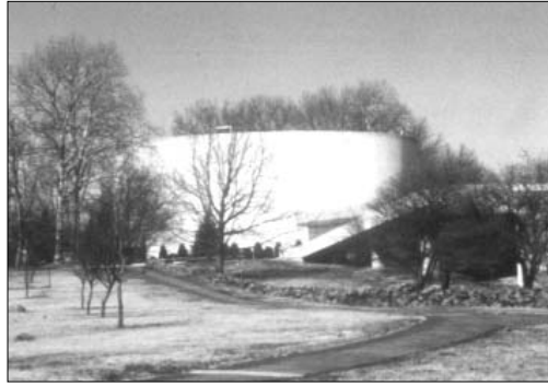
Cyclorama Building, Gettysburg. Designed by Richard Neutra. (Copyright Nathan Riddle.)
