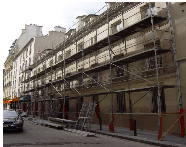
Reid Hall from the rue de Chevreuse entrance during renovations, 2006.
