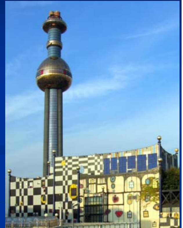
Waste to Energy plant in Vienna ( en.wikipedia.org )
