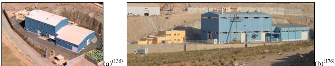
Figure 4.47 View of the MWI.
