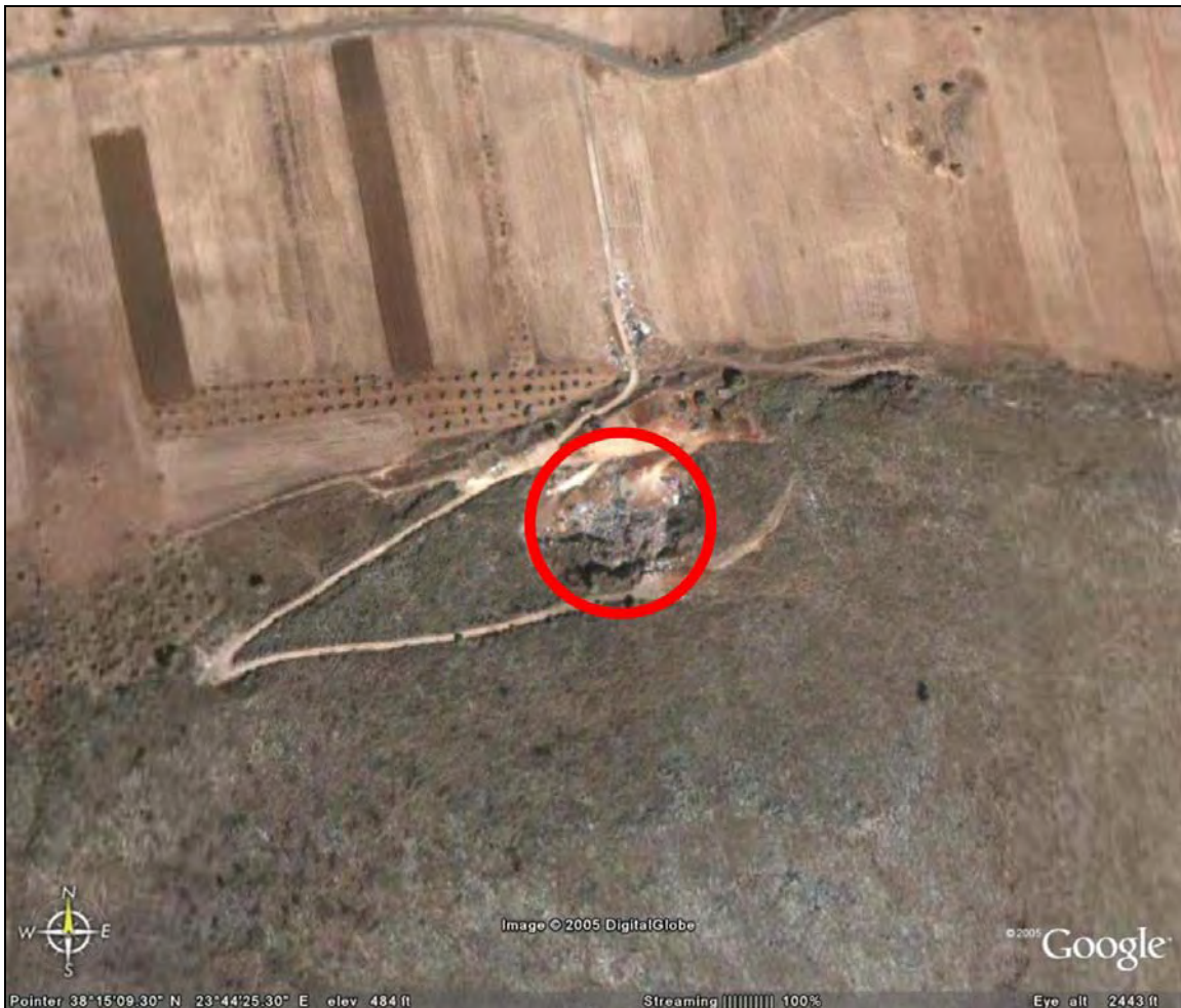
Figure 4.63 Aerial photograph of Avlona landfill (77) .
