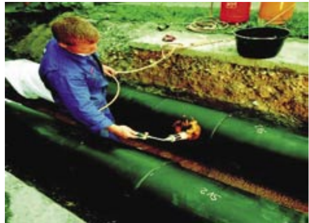
Figure 12.2 District heating mains being installed.
