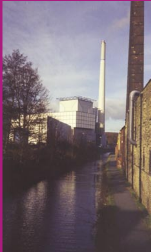
Kirklees Integrated Energy from Waste plant
