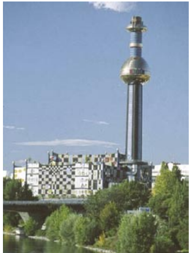
Innovative architecture used at the Spittelau EfW facility in Vienna
