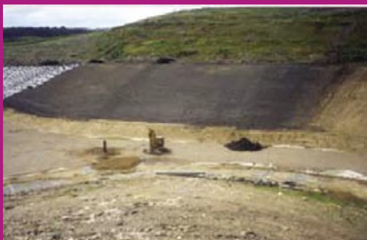
Cell construction at Burnhill landfill site
