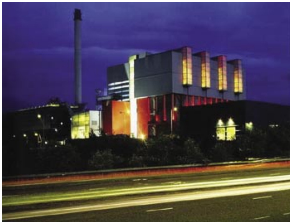
Tyseley Energy from Waste plant, Birmingham
