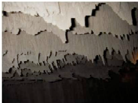
Figure 3-2. Accumulation of deposits on chloride trap [76]
