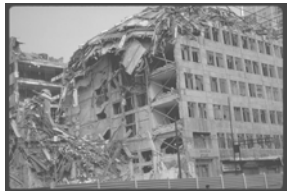
Mexico City, 1985 magnitude 8.1 estimated damage – $5 billion
