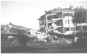
Pancake collapse of apartments in Goliaka, Turkey, 1999 Photo: Nano Seeber
