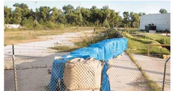
This 5-foot to 10-foot wall of sandbags and sheet piling runs south of Airline Drive to the Mississippi River levee near the airport. Surge water from the lake could pool along the river levee and pour over this barrier into Jefferson Parish and New Orleans, according to computer models.
