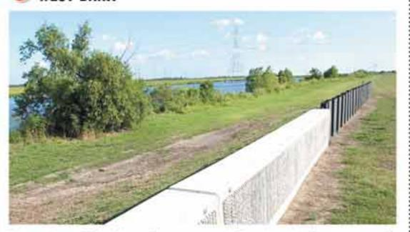
More than 60 miles of levees and floodwalls from east of the Harvey Canal to west of Lake Cataouatche – including this stretch of completed floodwall and yet-to-be-raised levee along Bayou Segnette State Park – are years from completion. Small hurricanes can push water from Timbalier and Barataria bays into West Bank neighborhoods.
