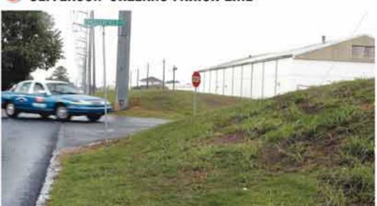
Chesterfield Street passes through a low levee from Monticello Avenue in Jefferson Parish into New Orleans near the city's water plant. Computer models indicate this is the likely spot for floodwater to enter the city from St. Charles and Jefferson parishes during hurricanes.
