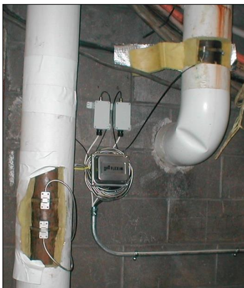
Figure 4-1. Flexim chilled water meter
