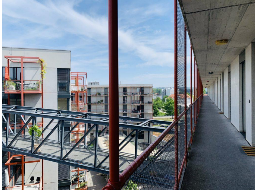
Zwicky Süd, view of court-yard and galleries. Courtesy of Bau-und Wohngenossenschaft Kraftwerk1
