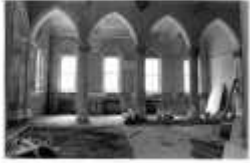
. 1The Chapel being reconstructed
