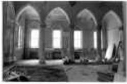
. 1The Chapel being reconstructed
