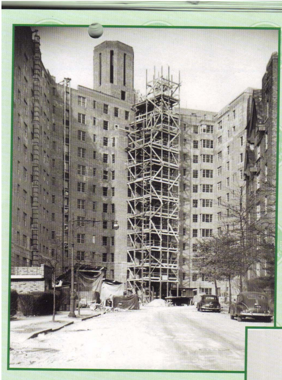
Bldg 8 under construction Winter 1950
