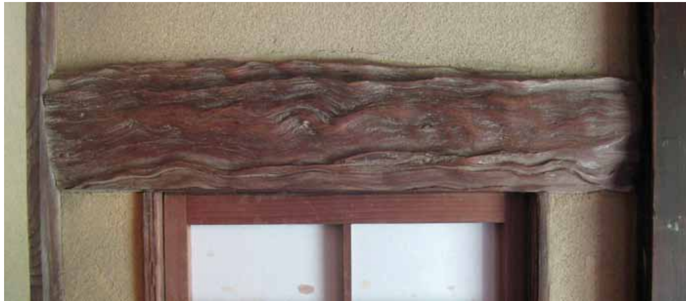
FIG. 8. Lintel of Chinese juniper above north window, visible in fig 1. Donation no. 54 in Mokuben kanjin , given by Akiyama Terue, chief priest of Mishima Shrine. Photo by author
