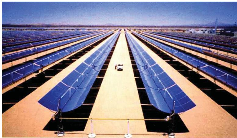
**Plate 12. Parabolic trough concentrators at Kramer Junction, CA.** The system, called the Solar Electricity Generating System (SEGS) installed at Kramer Junction in Mojave desert, California, starting from 1984. The SEGS system is the largest solar electricity generator set on the world. The total capacity is 354 MW.
