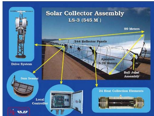
**Plate 11. Solar collector assembly of a trough system.** The axis of the parabolic troughs are aligned South-North. A tracking mechanism turns the troughs every day from East to West. The solar radiation is focused on the vacuum-tube heat collectors. The collectors heat synthetic oil to 400°C, then generates superheated steam to drive steam turbines. The highest efficiency on record was 20%.
