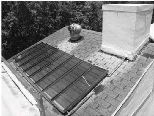
**Fig. 1.28. A Day-and-Night solar water heater in Florida.** From 1920 to 1941, more than 25,000 solar water heaters were manufactured and installed in Florida. After 70 to 80 years, thousands of them are still working. The photo, taken by the Author in Miami in August 2010, is a solar water heater installed in 1937. The insulated water tank is disguised as a chimney. Even with a broken glass, it is still working properly.
