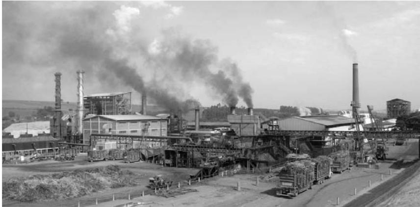
**Fig. 1.13. The Costa Pinto Production Plant of sugar alcohol.** The foreground shows the receiving operation of the sugarcane harvest, and in the right side of the background is the distillation facility where ethanol is produced. This plant produces the electricity it needs from baggasse left over by the milling process, and it sells the surplus electricity to public utilities. Courtesy of Mariordo.
