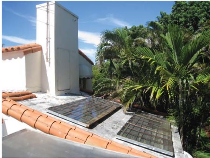
**Plate 15. Day-and-Night solar water heaters manufactured and installed in 1920s in Maimi.** The Day-and-Night solar water heaters could be very durable. After approximately 80 years of operation in violent weather conditions in south Florida, thousands of such solar water heaters are still working properly today. The secret is its simplicity and complete absence of moving parts. Photos taken by the Author in August 2010, Maimi.
