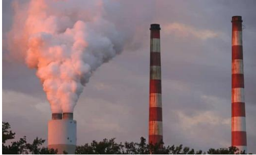
The coal-fired Morgantown Generating Station in Newburg, MD.
