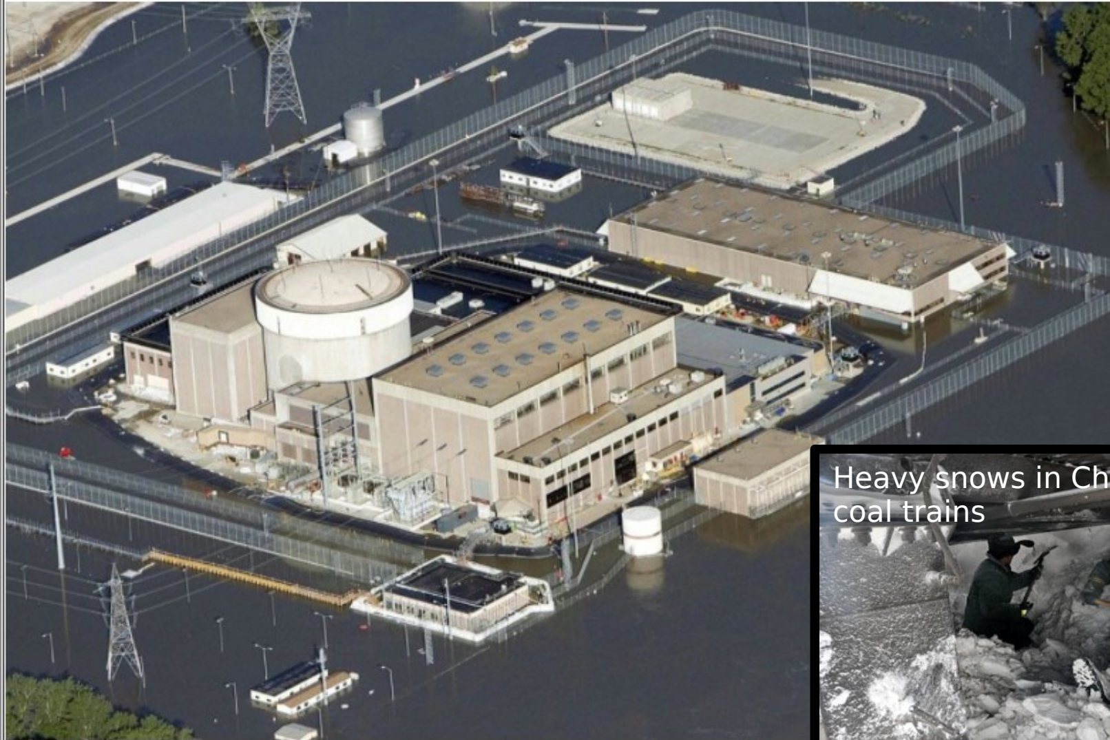
Fort Calhoun Nuclear Power Plant, about June 18, 2011
