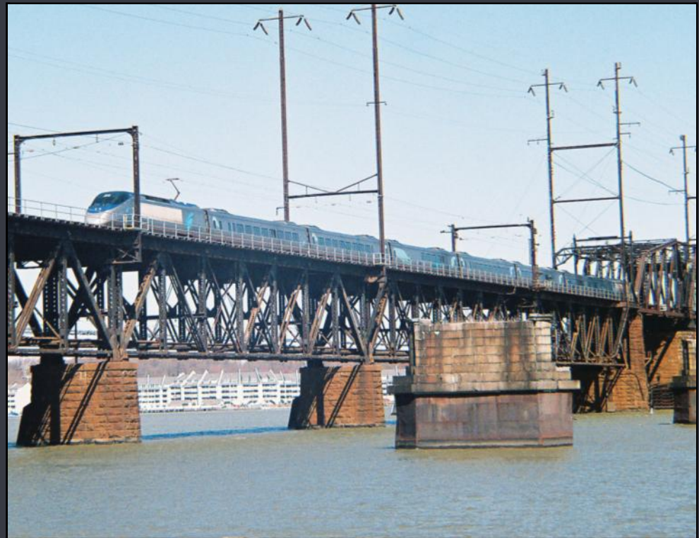
The Susquehanna River Bridge in Maryland was built in 1906.
