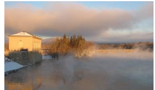
Ashokan Reservoir, a component of the New York City Water Supply System
