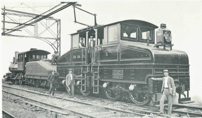
95 TON ELECTRIC LOCOMOTIVE, BUILT IN 1895 BY GENERAL ELECTRIC COMPANY
